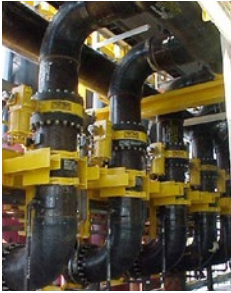
Bondstrand GRE piping systems inside the hull
