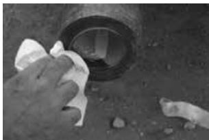
Clean excess paste from mold
