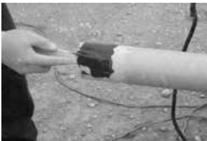
Apply paste to pipe
