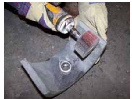
Sand the inside surface of the saddle
