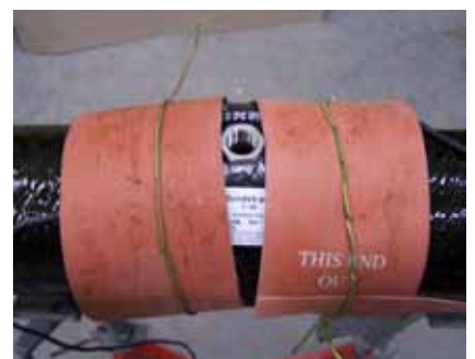
Use NOV FGS heating blanket for heat cure
