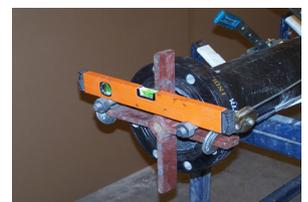
Photo 17 - Check alignment of bolt holes
