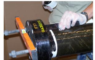
Photo 10 - Remove excessive adhesive
