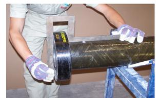
Photo 9 - Check alignment of flange face
