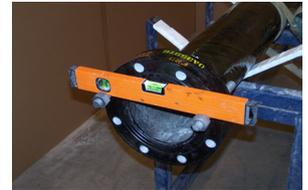
Photo 7 - Check bolt holes alignment
