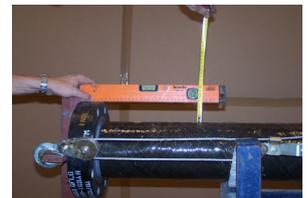
Photo 16 - Check alignment of flange face
