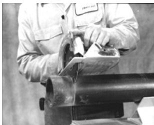
Sawing the pipe
