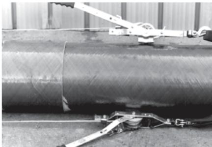
If the straps slip on the slick pipe or fitting surface, emery cloth placed between the strap and the pipe or fitting will increase the frictional resistance to slipping. Abrasive powders such as Ajax or Comet may also be used under the straps to help prevent sliding.
