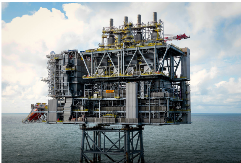
Figure 1. The Clair Ridge platform, a state-of-the-art facility where BP will begin recovery of 640 million bbls of oil and deploy their LoSal® EOR technology for the first time.
