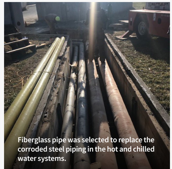
Our Red Thread piping was selected for the 4,000 ft. of chilled water supply and return.
