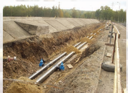
Bondstrand 2000 with Quick-Lock adhesive-bonded joints is used for various firewater, sewerage and cooling water lines.
