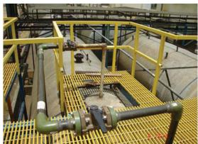
Application: Sulfuric acid in operating conditions of 2% to 6% and sodium hydroxide at 98%. The operating
