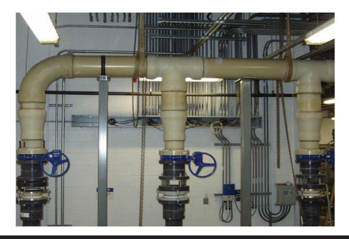
Application: Transport of acid waste streams from the process facility to the on-site wastewater treatment system
