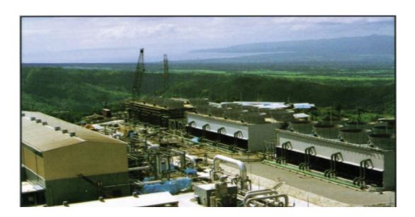
Application: Condensed geothermal steam cooling tower supply and return lines operating at 165°F at the world's
