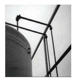
Application: Lines Carrying 78% sulfuric acid and hydrochloric acid used for the production of chemicals for the
