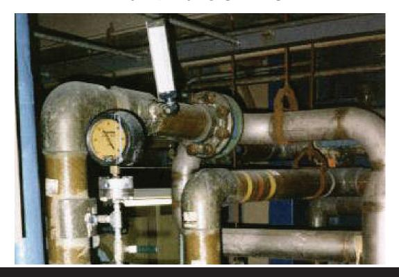
Application: Paint is carried from a mixing area to an electro-coating vat and through a recirculating system. Paint
