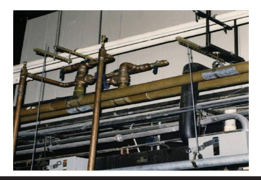
Application: Chilled and hot water lines for heating and air conditioning system update
