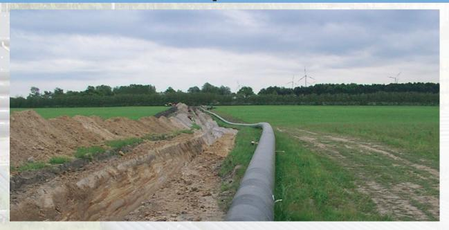
In 2001, NOV Fiber Glass Systems B.V. secured the contract for an 18 inch GRE brine transport line with a working pressure of 20 bar with a total length of 54 km. Leading energy supply company EWE (Elbe Weser Ems) planned to create four caverns, at a depth of 1200 meters, 450 meters high and 100 meters in diameter, with a volume up to 700.000 m³ each in the underground salt layers of Rüdersdorf, located some 30 km east of Berlin. The caverns were created for storage of natural gas.
