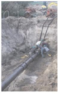
aid of laser-guided excavators. This approach of trench preparation often resulted in trench depths of more than 5 meters.
