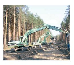
the trees were covered with protective material. Thrust boring was used in sensitive areas and biodegradable hydraulic oil was used in equipment and all types of waste were disposed of properly. A battleground where the Soviet Union army fought to take Berlin in the last days of World War II was the area in which the pipeline was installed. Before excavation work could begin, the route was checked for live ammunition to ensure a safe installation. Several pieces of World War II scrap were found.
