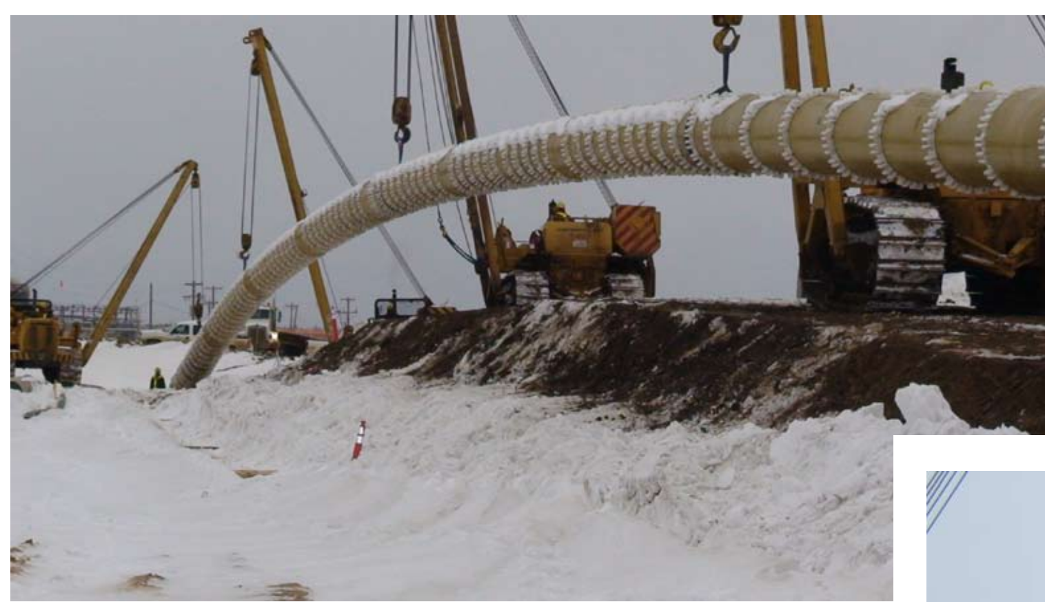
In April, the Team set the record with their 640 metre 36" GRE pull under the Muskeg River. A month later, they broke their own record!
