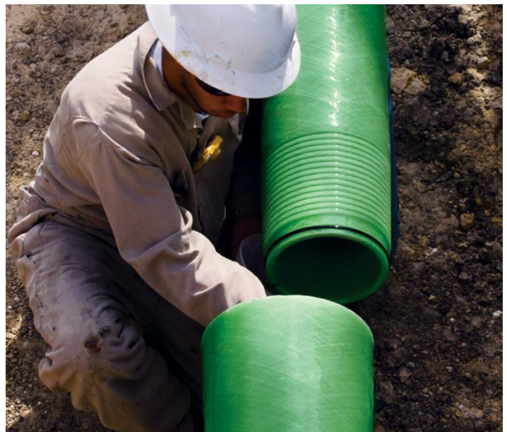
8 inch, 2,500 psi STAR Super Seal pipe with SS HP connection
